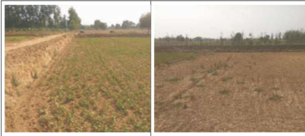
Figure 20-6: After Backfilling Topsoil Closed Borrow Area
