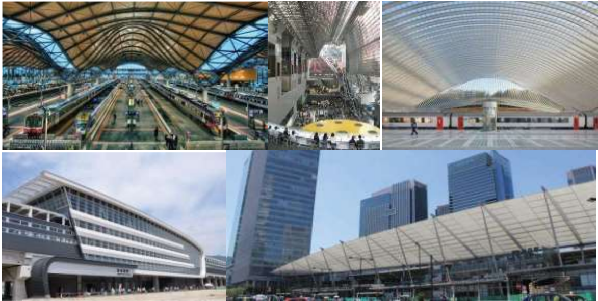
Figure 20-9: Image of Station Buildings
