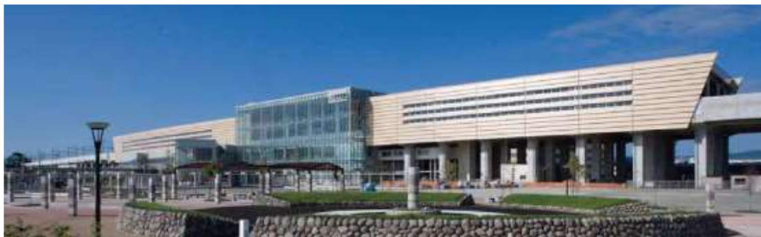
Figure 20-10: Façade Image of the SilverLine Station
