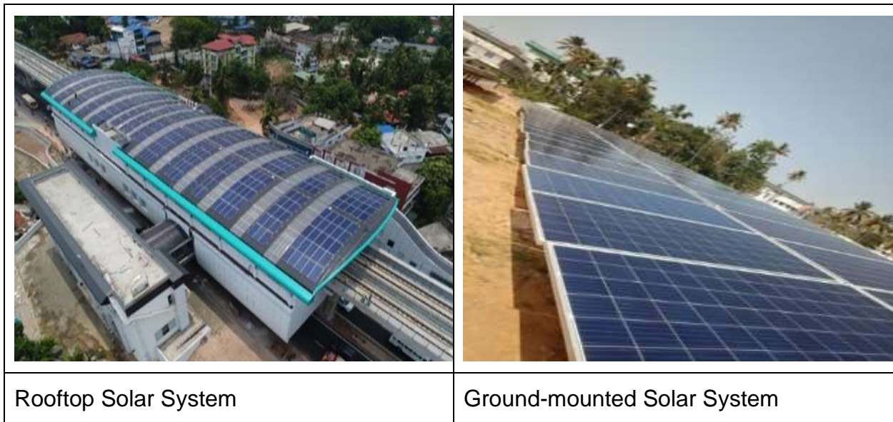
Figure 20-15: Mounting arrangements of solar panels in roof top and Ground
