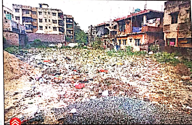
The water body has been filled up apparently to carry out constructions there
